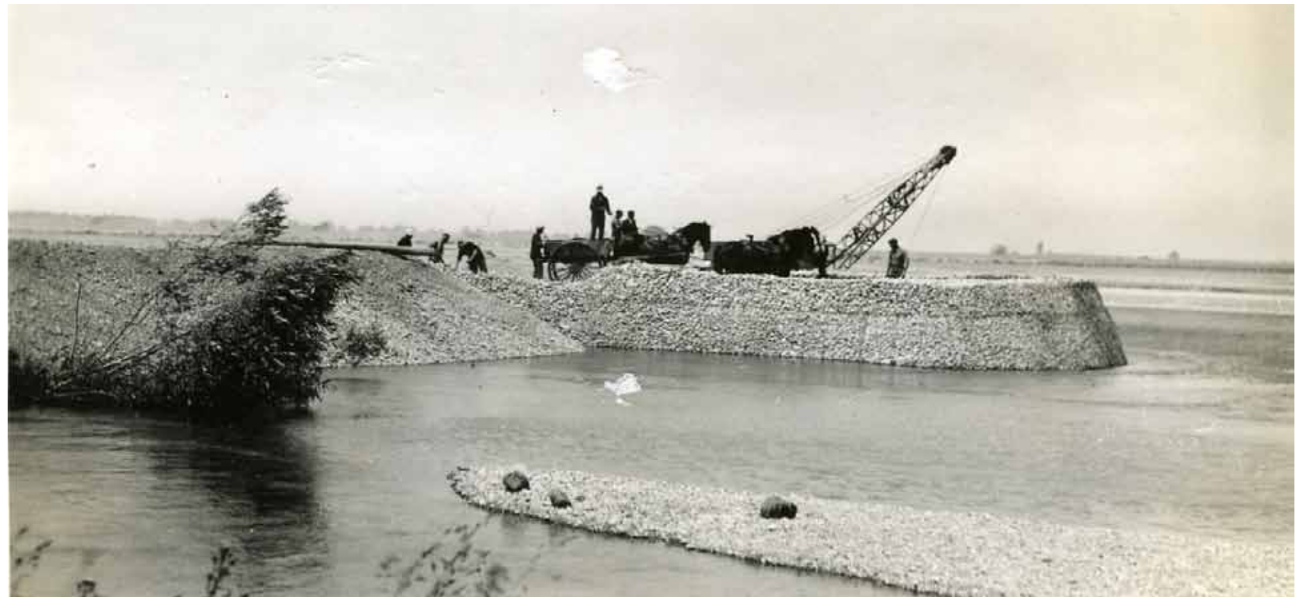
Early stopbank construction on the Waimakariri River
