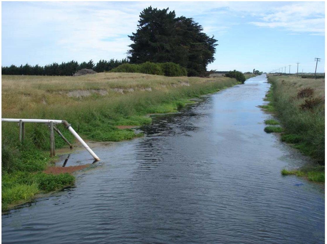
Figure 5: Halswell Canal at Duck Pond Rd. This canal copes well with long term drainage needs, but the capacity is not adequate in all sections to contain stormwater runoff.
