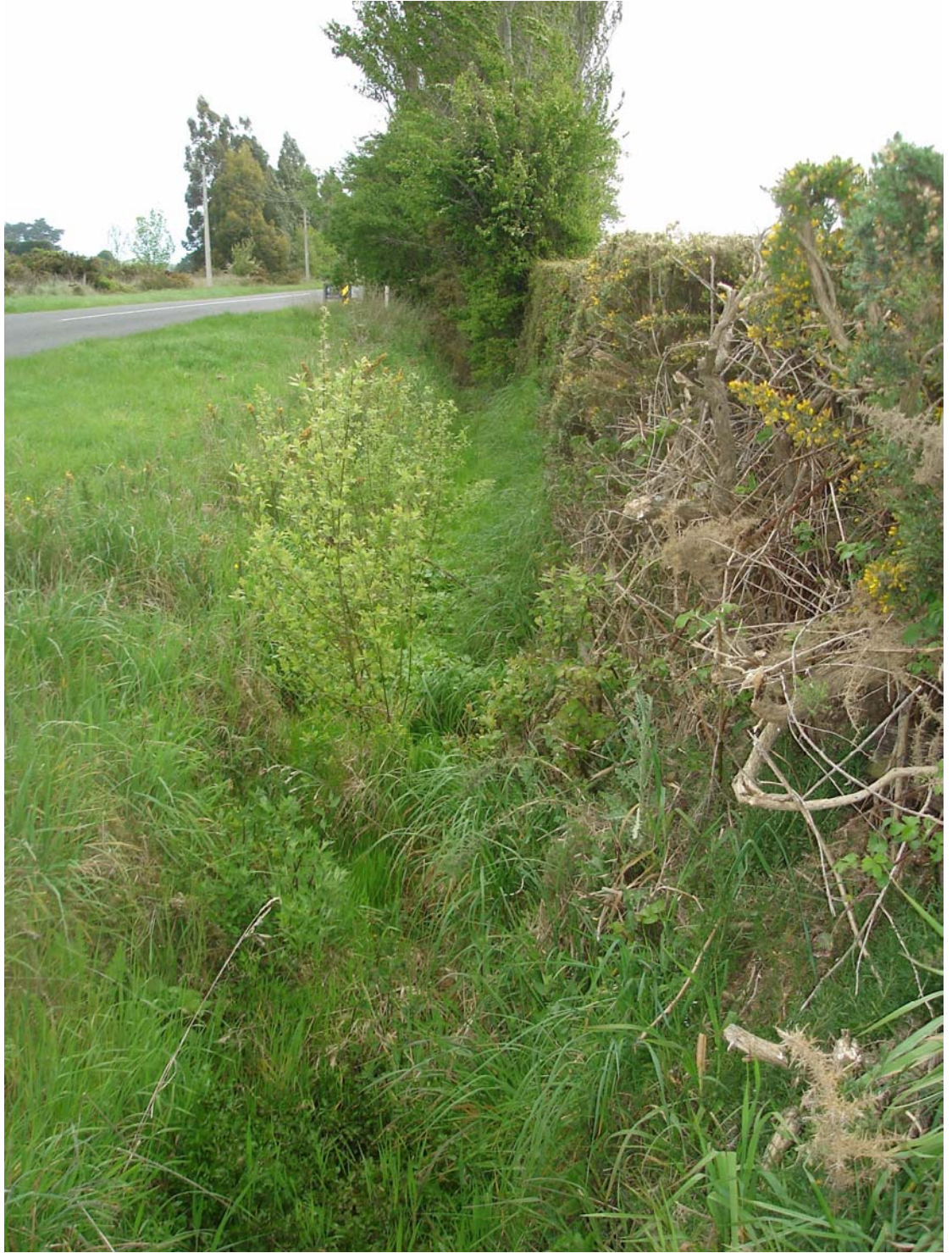
Figure 10: Overgrown drain by Lake Road. This is an example of a drain whose capacity and performance could be improved by more frequent cleaning
