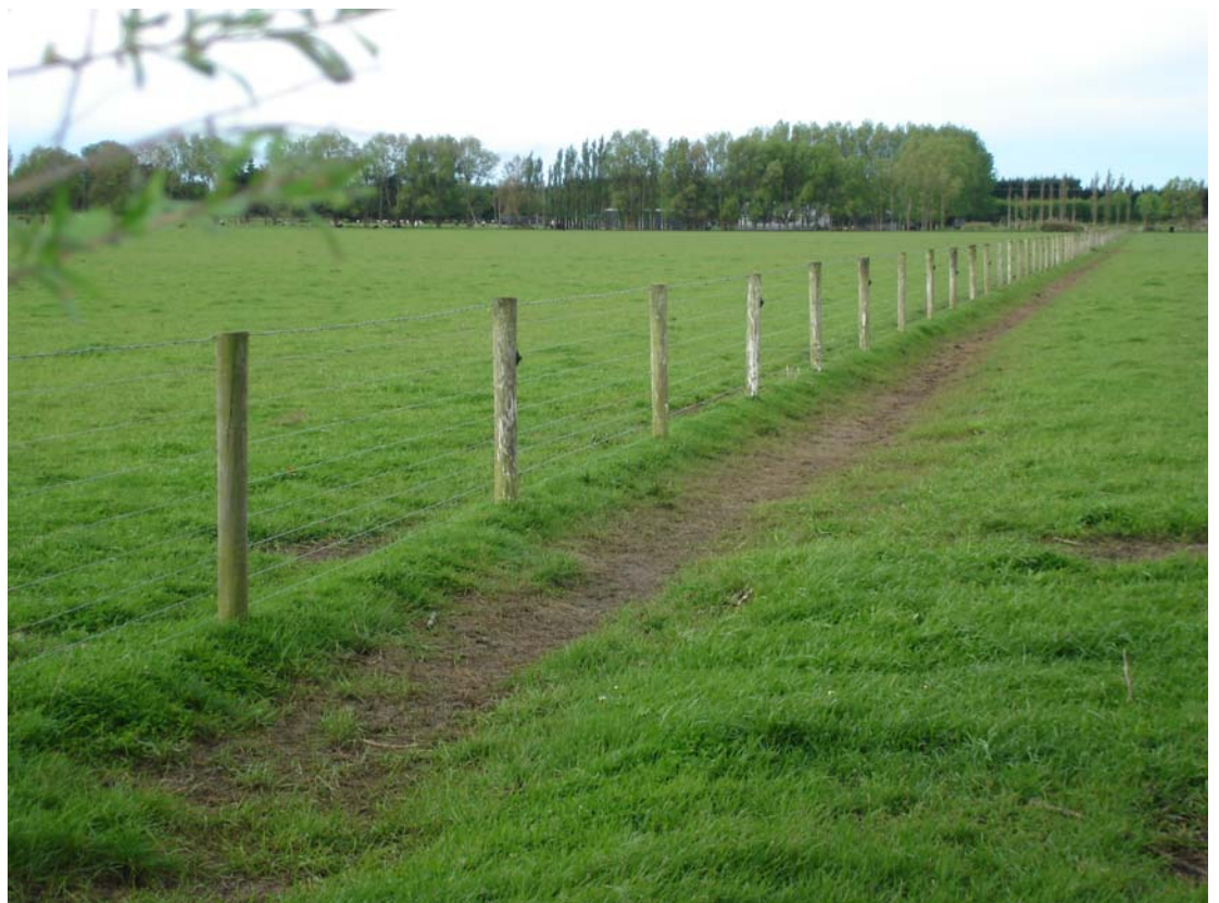
Figure 9: Swale drain alongside fence. This is an example of an unobtrusive drainage improvement that could be suitable in some locations
