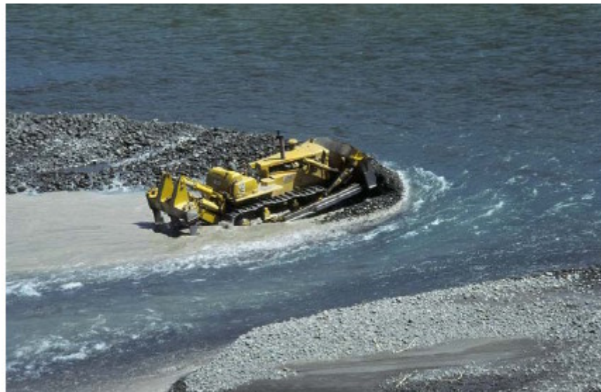
Figure 14: Bulldozer constructing diversion works in Hurunui River
