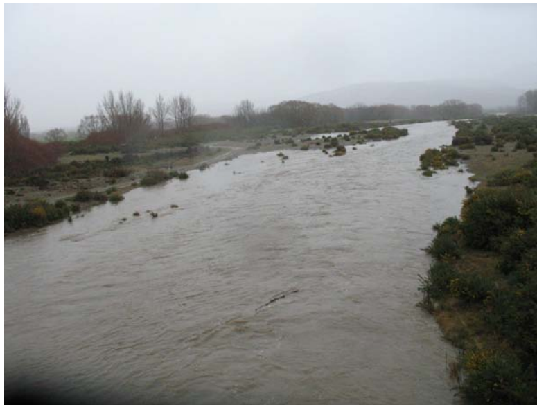
70 cumecs and rising. Flood flows in the Hakataramea River July 31- 2008. The last significant flood in the Hakataramea River was in August 2000.
