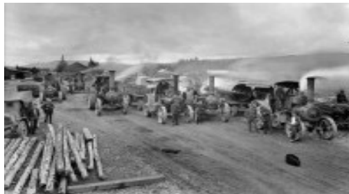
(Fig 2.)Traction engines await loading in Coalgate, to transport fluming to Lake Coleridge.
