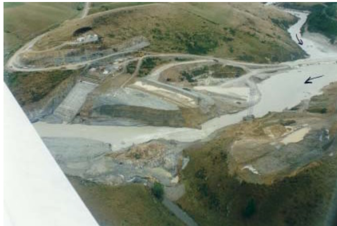
(Fig 6.) The Opuha dam after the breach.
