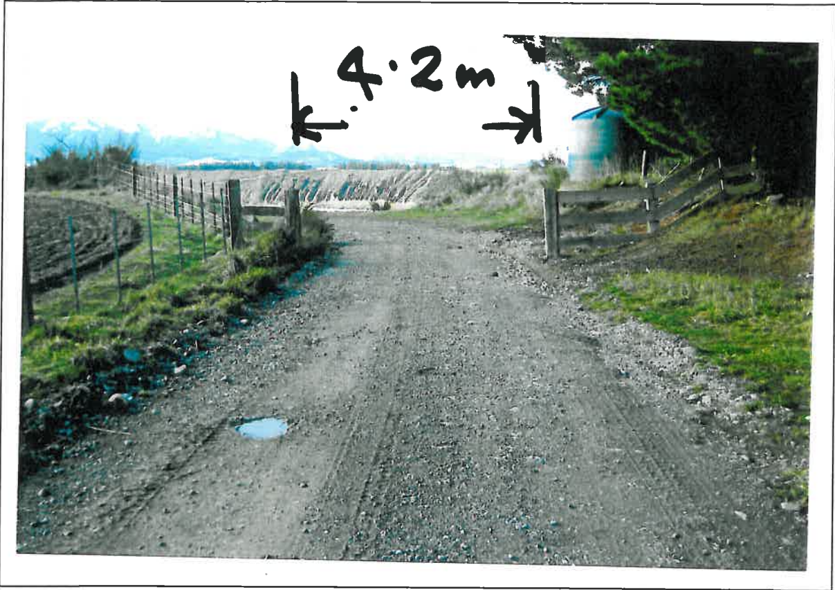
Entrance to steep decline and hairpin bend. 4.2 metres between posts from this point road drops 50m to river flat
