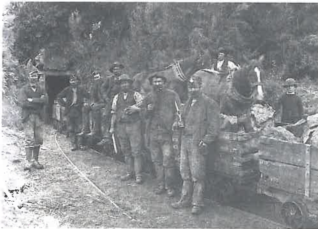
Entrance to Homebush mine
