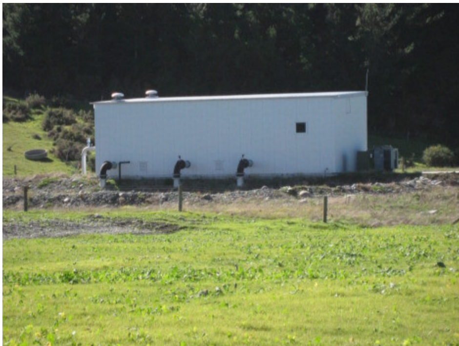
Closeup of the pump shed near Sleeman`s Rd
