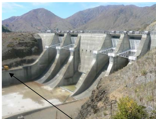
Picture 4: Spillway at Benmore Dam (note the yellow truck on the left which gives size context)
