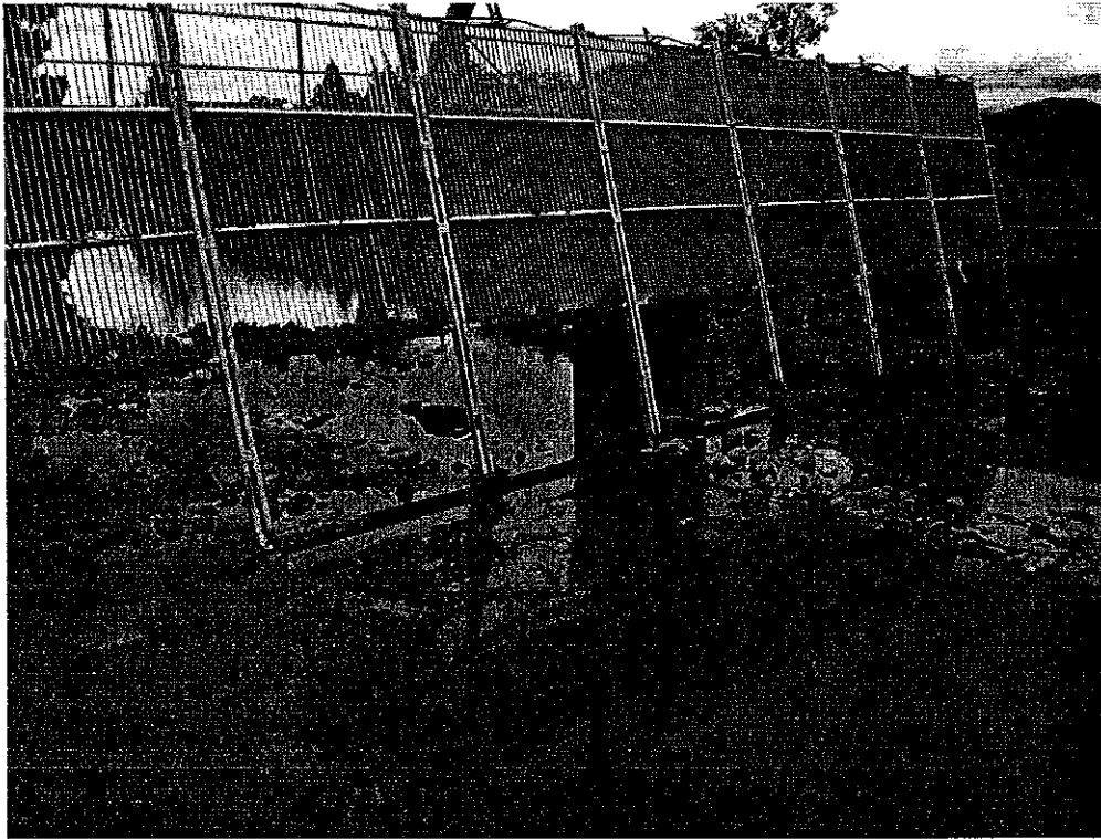
Figure 3: Salmon barrier (in a raised position) and concrete lined channel.
