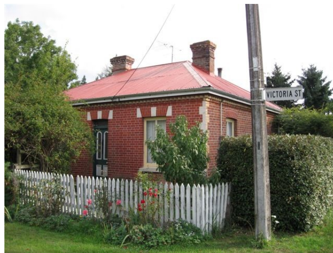
Early Glentunnel Brick Cottage.
