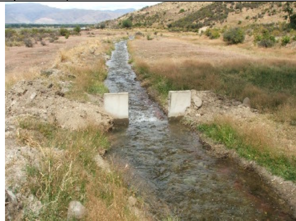
Control structure in race
