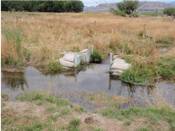
Diversion structure allowing flow to continue down Wairepo Creek
