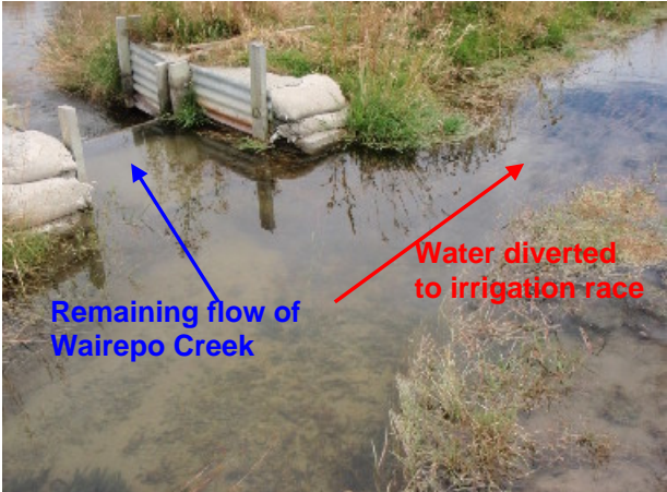
Diversion structure at intake, currently no water meter or flow gauge
