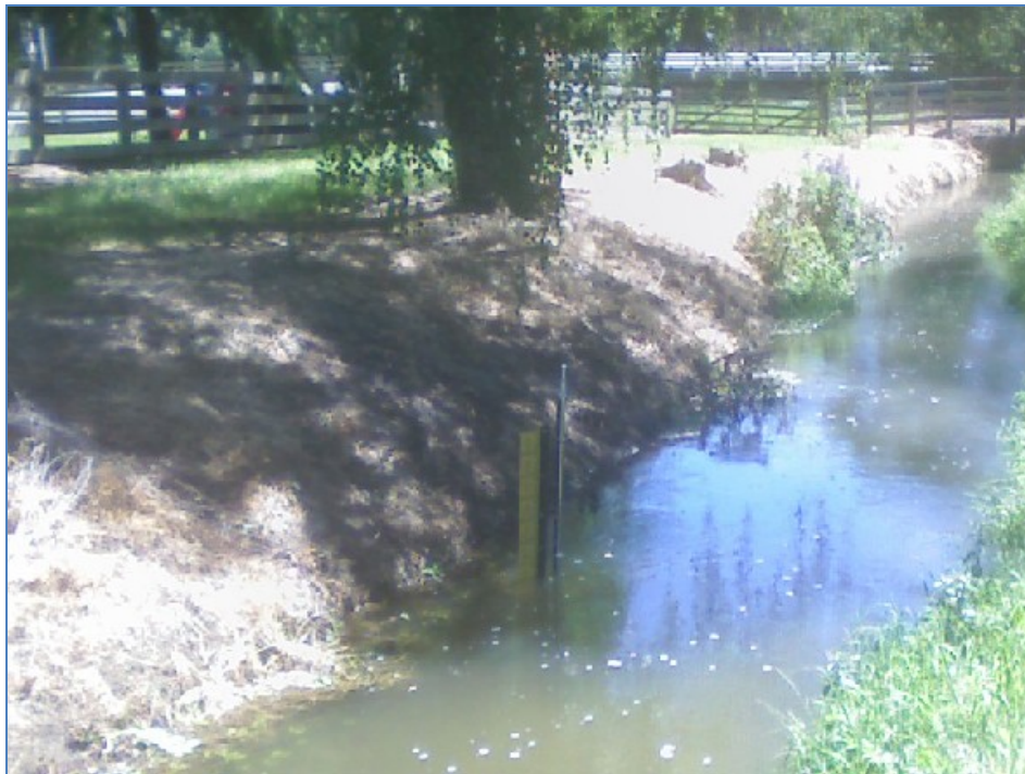
Photo 1: Haldon Station discharge channel below settling ponds. Flow in race 362 litres per second. Provided by Richard de Joux, 21 July 2009.
