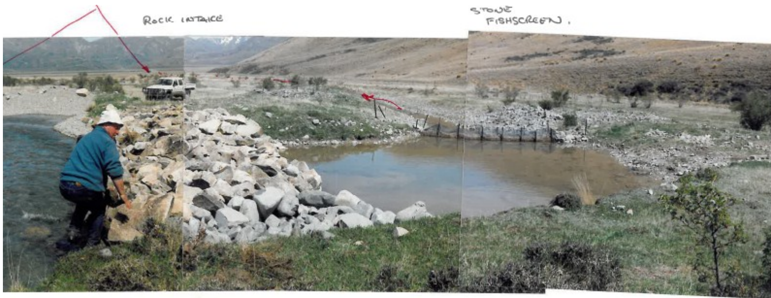
Rock gallery at intake with settling pond and stone fish screen / weir
