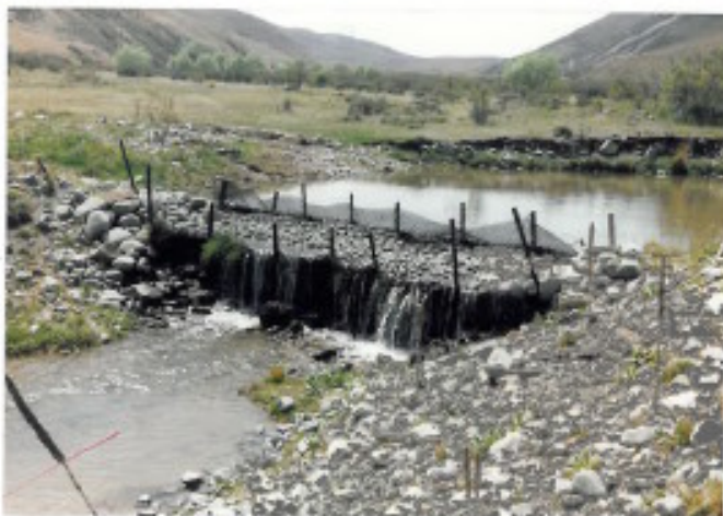
Rock gallery at intake with settling pond and stone fish screen / weir
