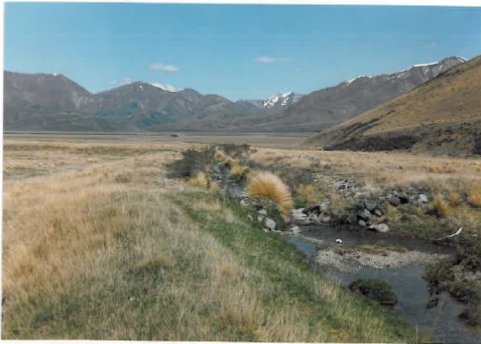
East Branch race downstream of intake
