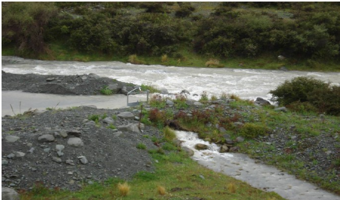
Photo 2 – close up of gate on diversion channel
