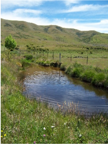
Buffer pond at intake site
