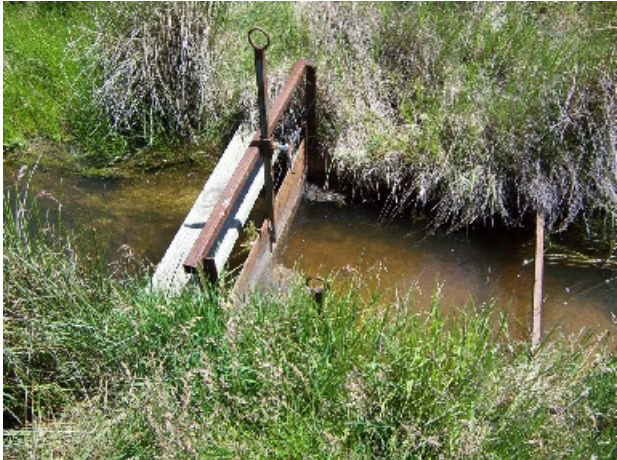
Control gate at intake
