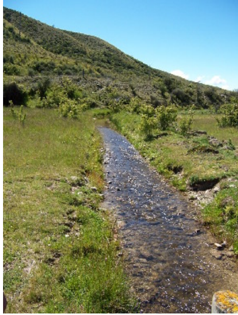
Diversion race after passing through intake gates
