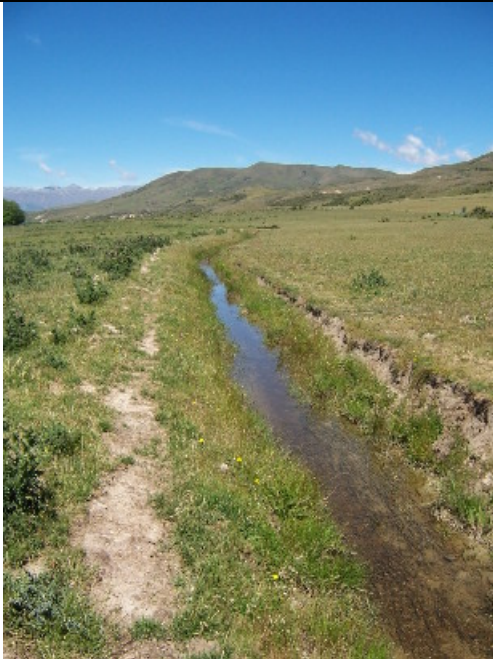
Diversion race providing stock and irrigation water
