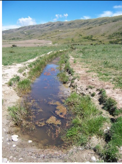
Diversion race providing stock and irrigation water
