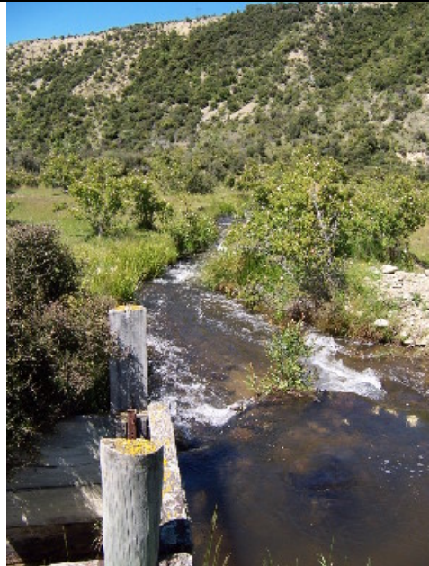
By-wash at intake gates back to Quail Burn
