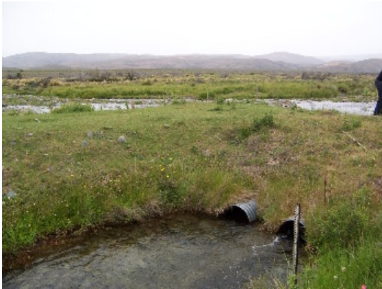
Intake pipes in Otamatapaio River
