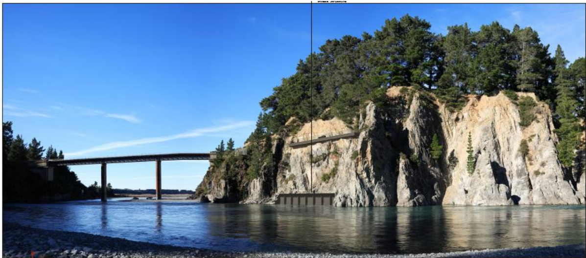
Photo point (13) At 5.7 Years - Lower Waimakariri River Intake Structure
