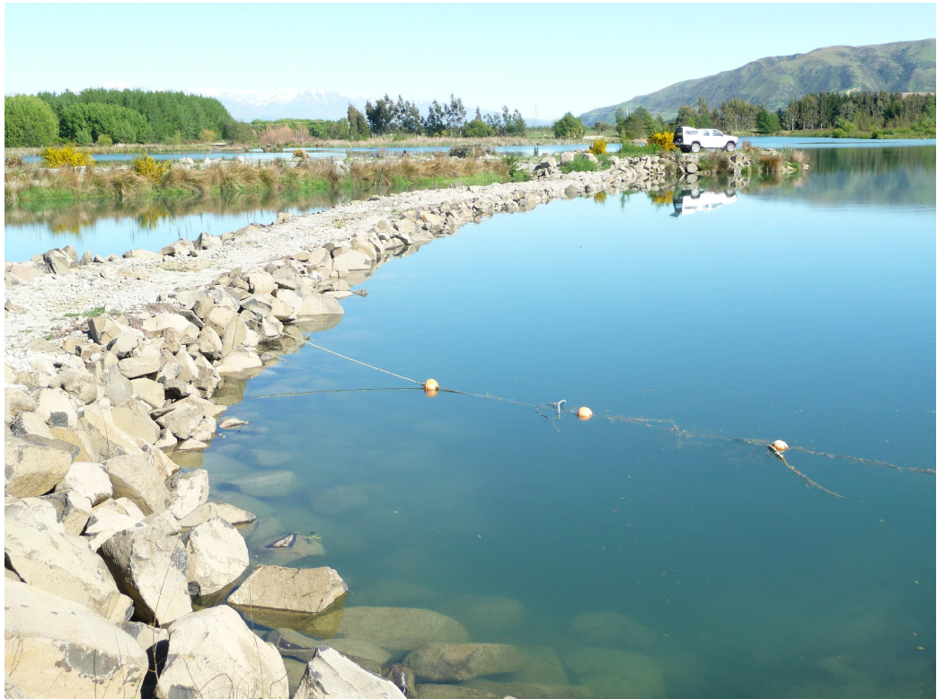
Figure 1: Boulder bank at intake to North Otago Irrigation Company Scheme
