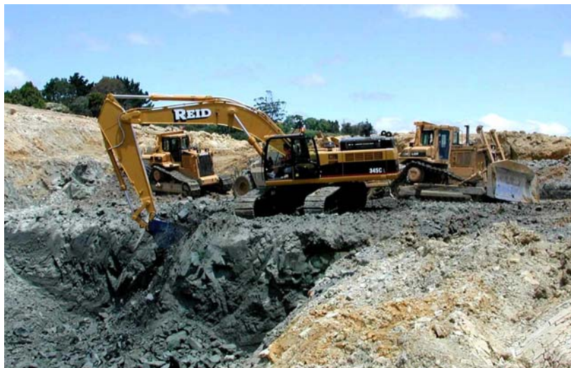
FIGURE 6. EXCAVATOR LOADING SCRAPER
