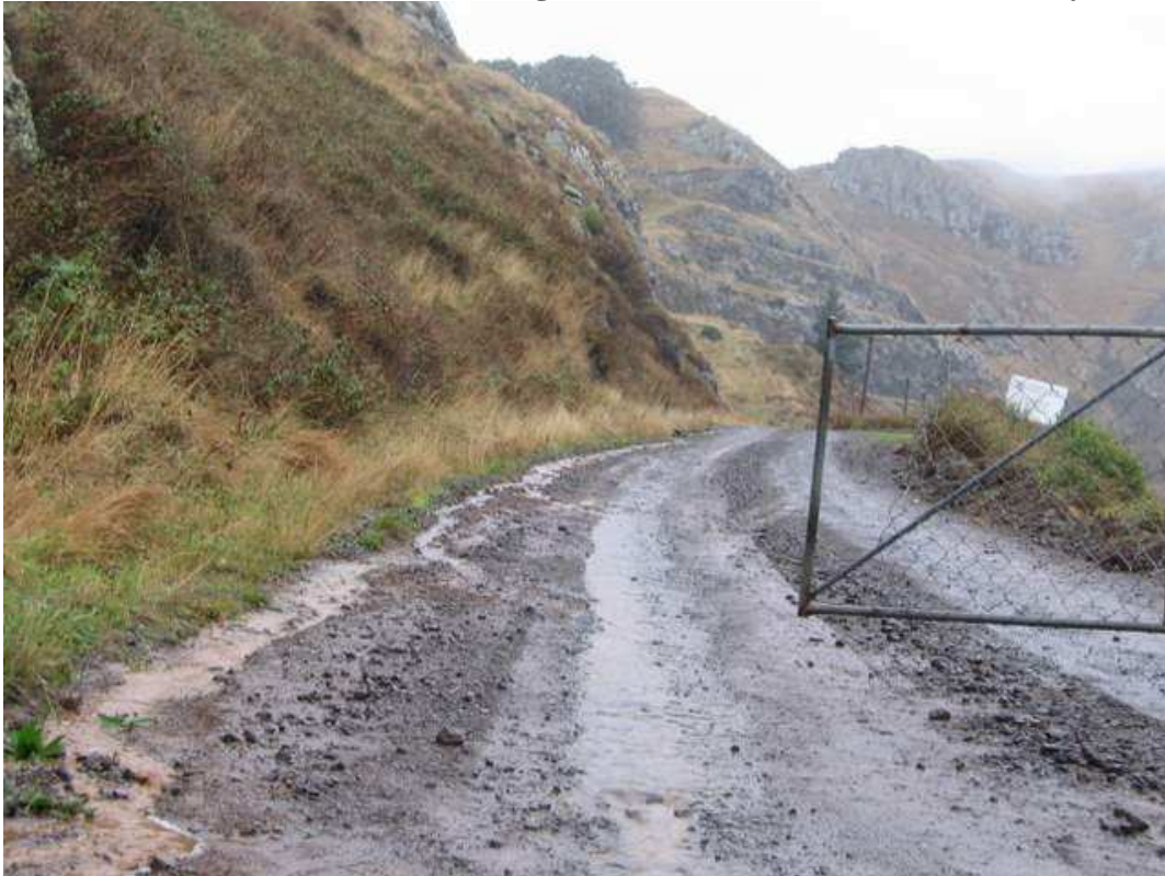
Photo 5: Old Sumner Road showing Clean Runoff from Road and Dirty from Hillside
