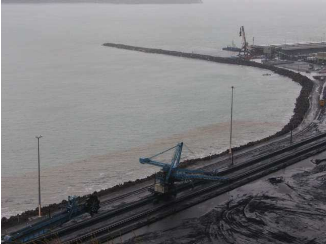
Photo 7: Western Outfall Discharge into Bay
