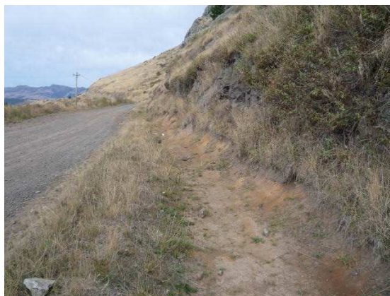
Figure 6 – Photograph of the Drain alongside the Haul Road
