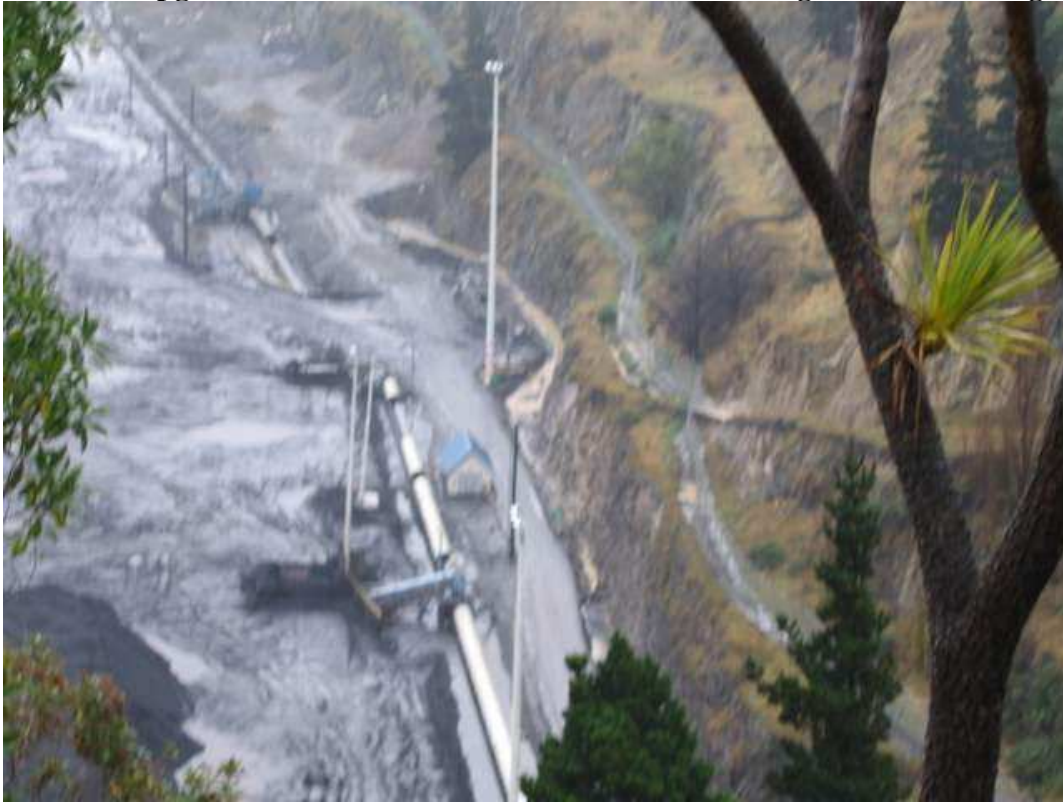
Photo 3: Upgradient Western Drain in Coal Yard Showing Loess Colouring
