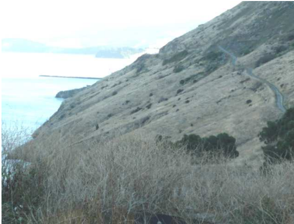
Figure 2 – Old Sumner Road Section of Haul Road
