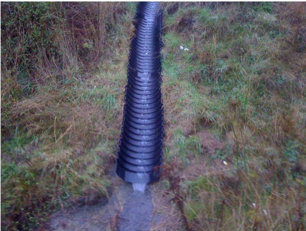
Photo 6: Clean Runoff from Sumer Road
