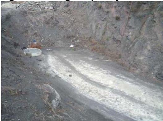
Figure 1 Existing Sump Entry to Western Outfall
