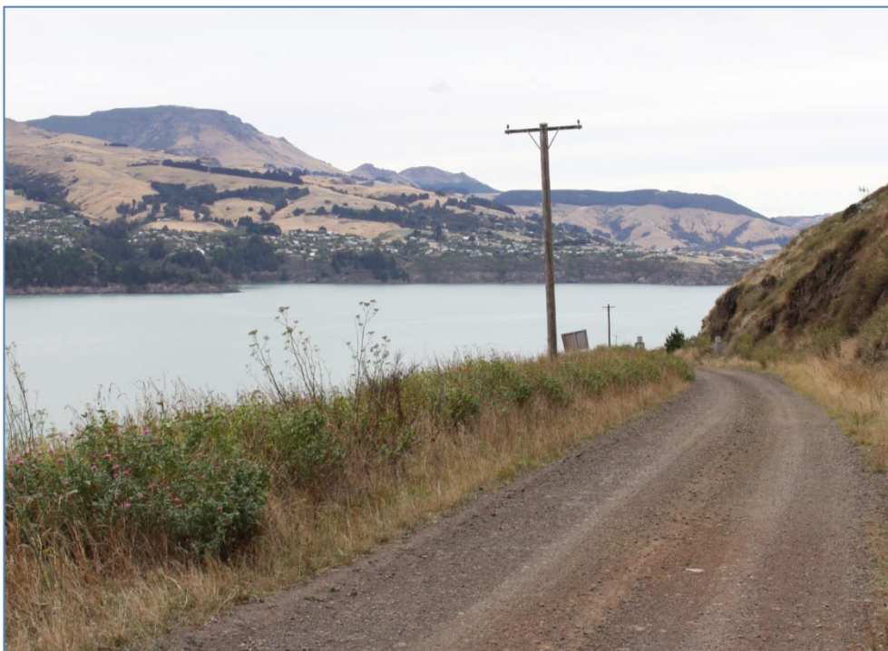
Photo 4. Existing haul road. Note dominance of exotic vegetation.
