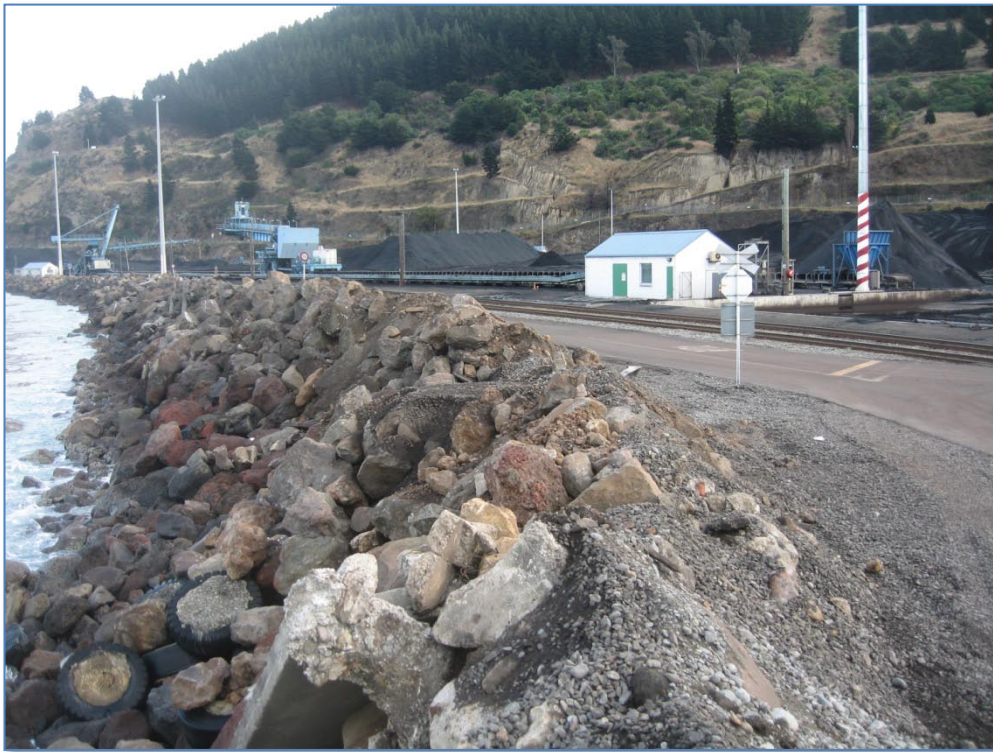
Photo 6. Coal yard at Te Awaparahi Bay, with seawall on left.
