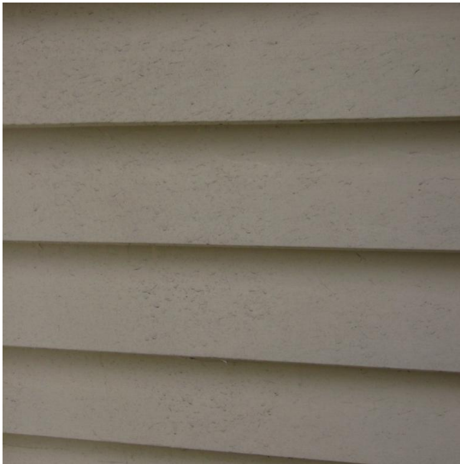
Figure 2: Examples of dust accumulation at 6 Randolph Terrace.
