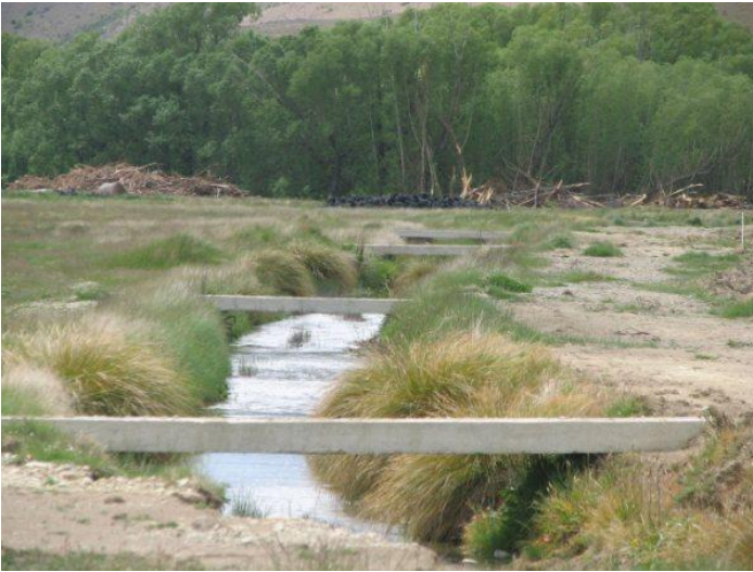
Photo A: Bridges where the pivot crosses the creek
