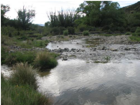
The intake from the Quailburn that will be upgraded
