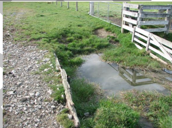
Another culvert where stock have access to water and have caused some erosion
