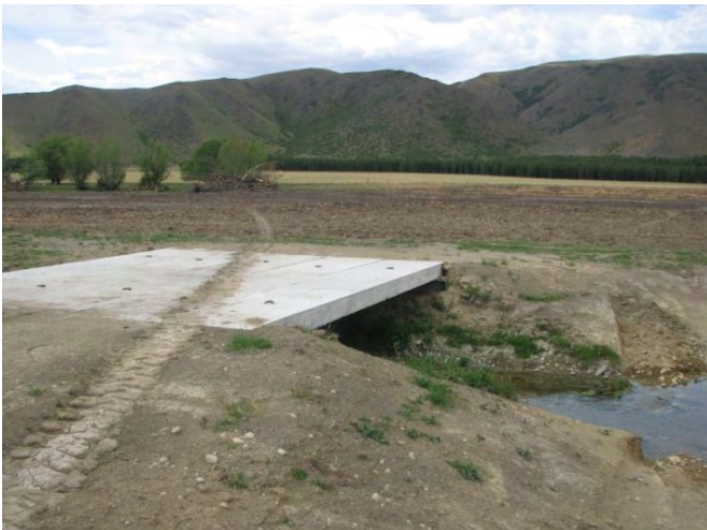
Photo B: Vehicle/Stock Bridge where the pivot crosses Wairepo/Spring Creek. Once finished the bridge will have a gate installed and a fence either side.
