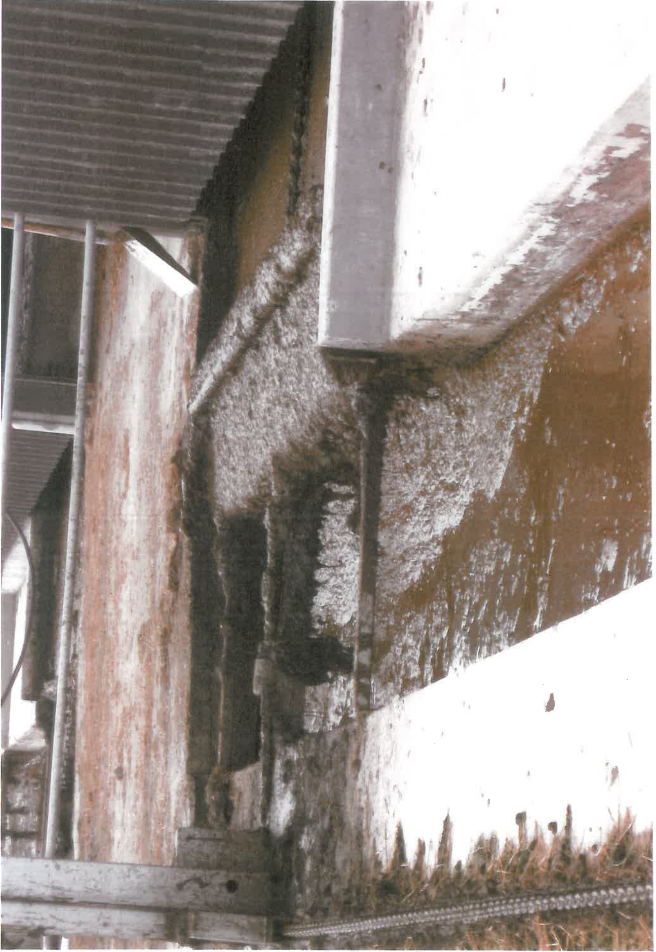
Photo 7: Effluent scraper discharging effluent into a drain at the end of the barn
