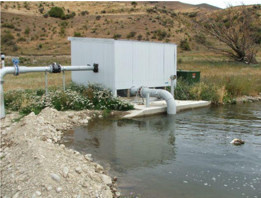
Photo 2: Existing pump station
