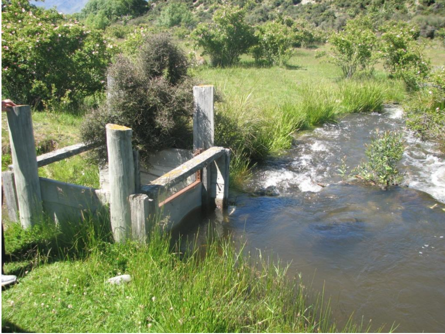
By-wash (discharge) at intake
