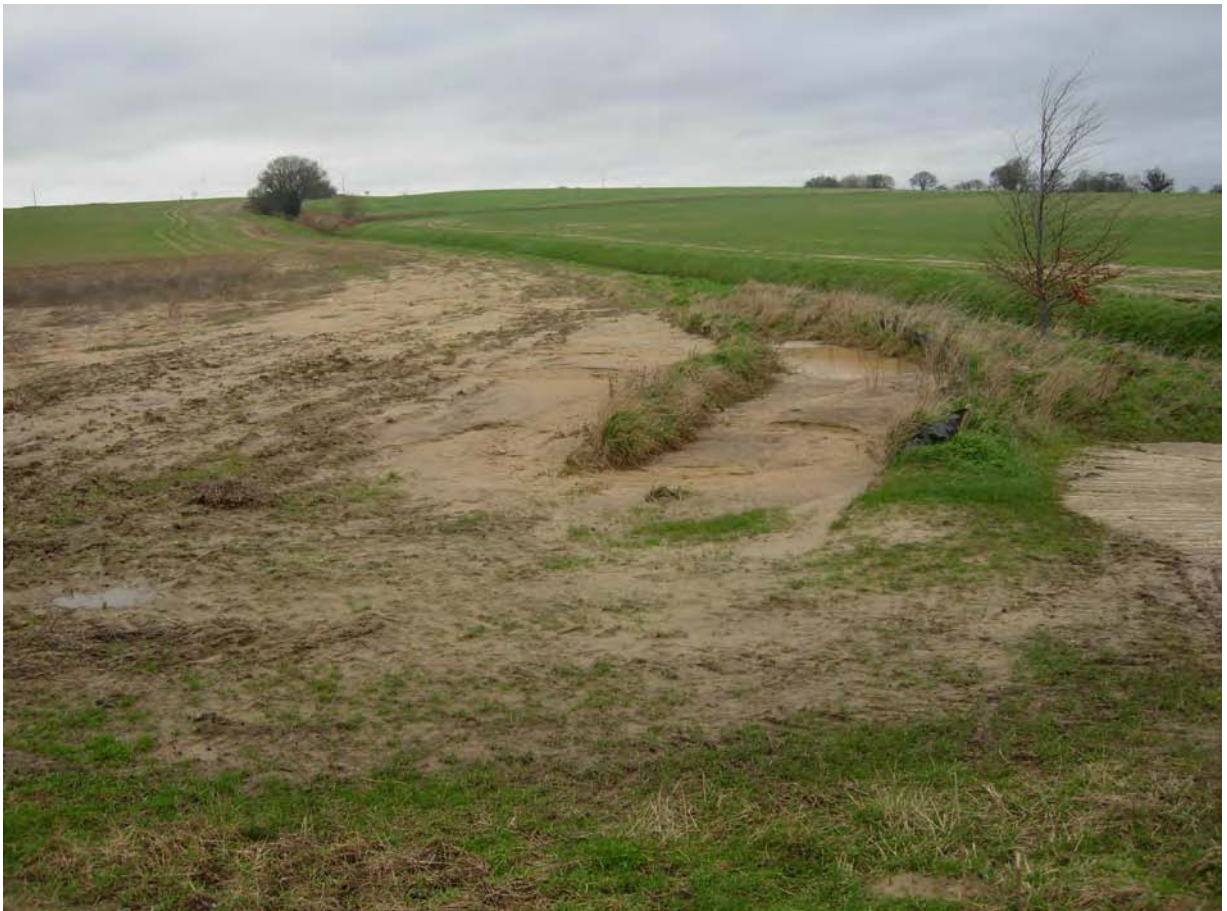
Figure 10 Field sediment trap
