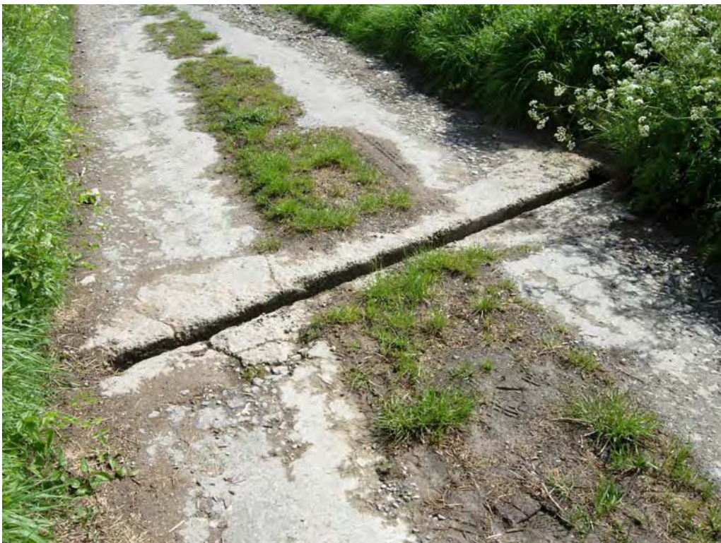
Figure 13 Cross drains on track for water removal
