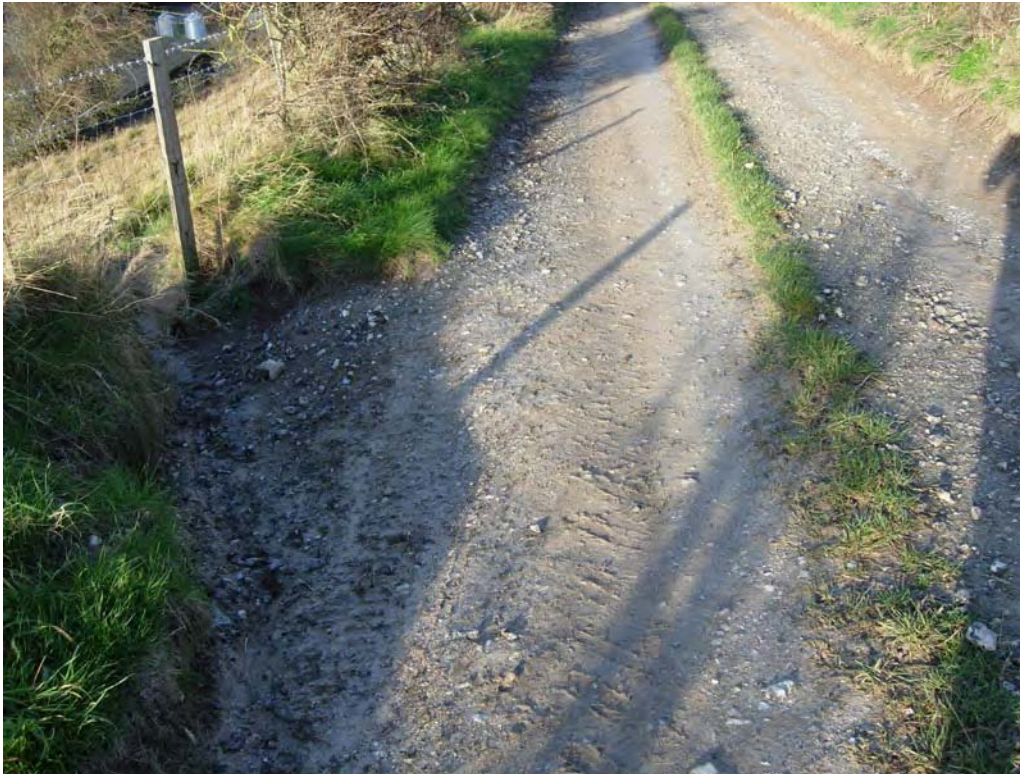
Figure 13 Cross drains on track for water removal
