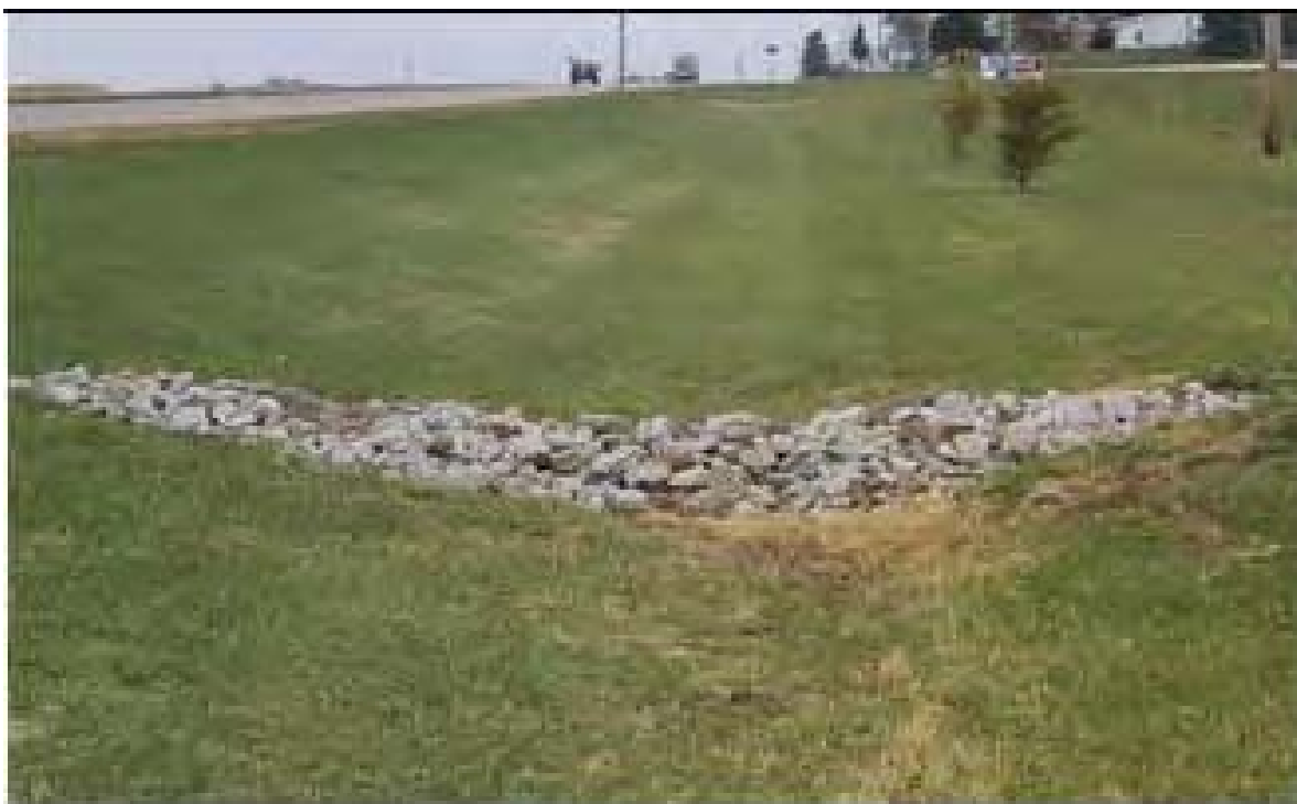
Figure 9 Swale with check dams to manage runoff
