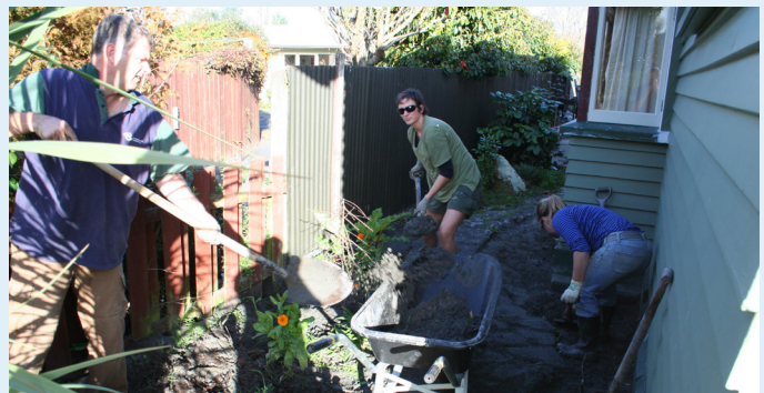
Kate and her team digging liquefaction after the June 2011 earthquake
