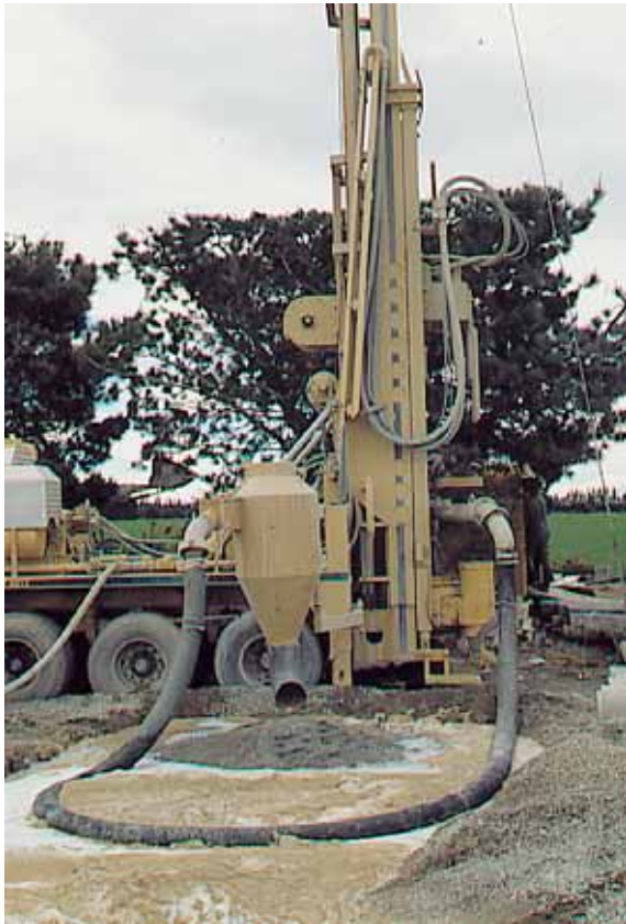
Dual rotary drilling rig in action.
