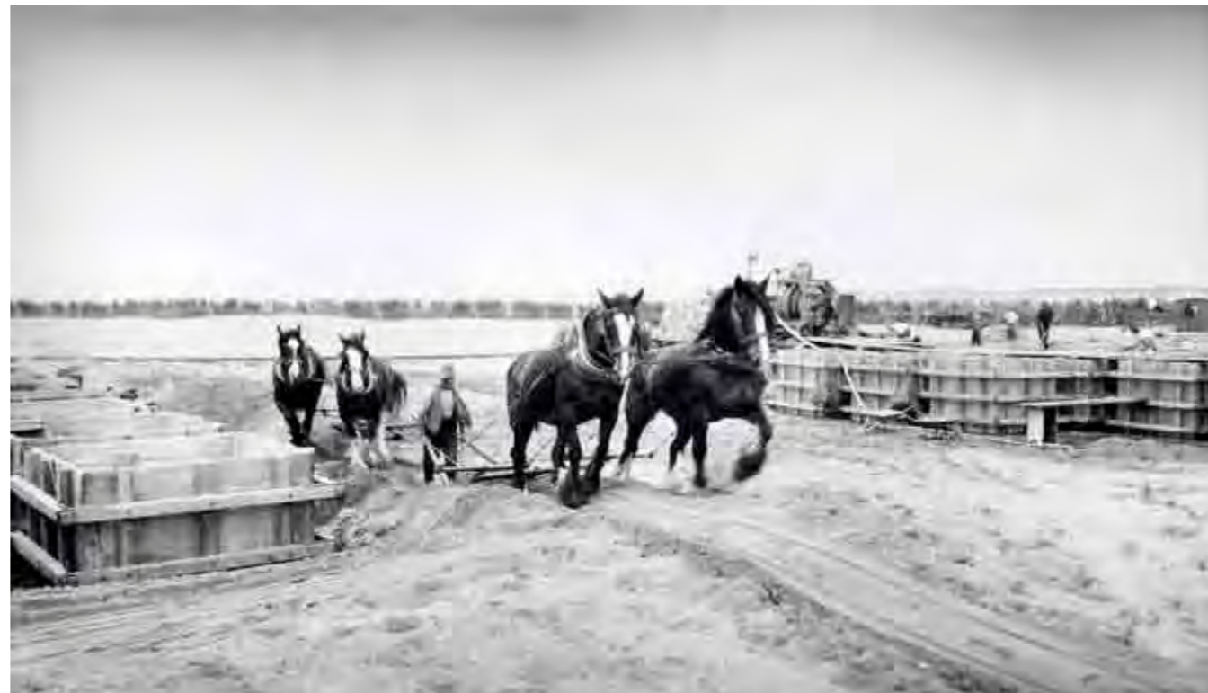
Early flood protection works
