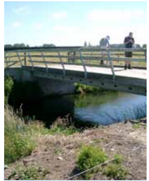
Bridges and culverts keep stock out of natural waterways.
