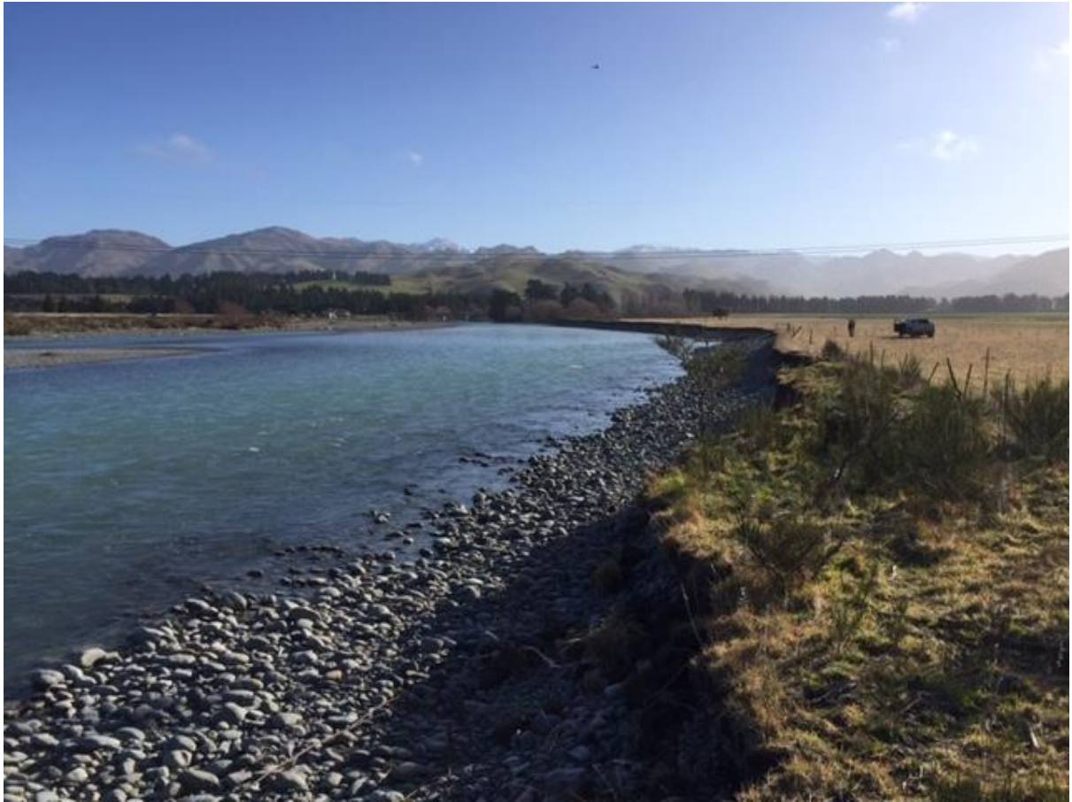
Photograph looking westwards, upstream, at scour of true left bank at upstream location. Note power lines across Waiau River at this site. AIC Scheme on left bank and Twin Bridges in the distance.
