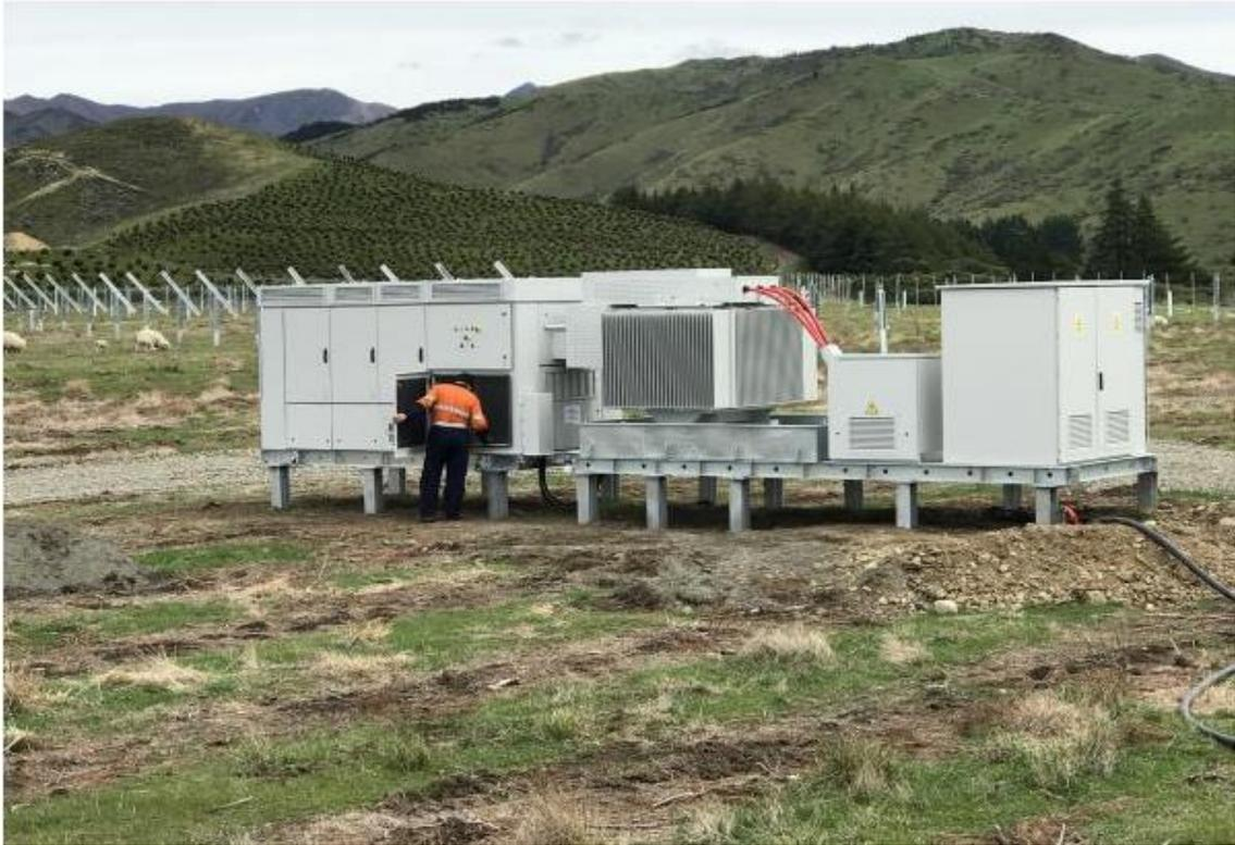
Figure 4: Photograph of HEMK MV skid gen 3
