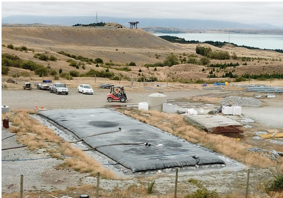
Figure 2 Geofabric dewatering bag/cell used at Tekapo by Mt Cook Alpine Salmon.
