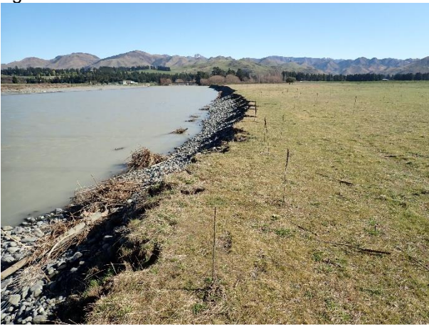
Figure iii. Upstream-most proposed ATP reach. Less erosion than downstream, but still present. No signs of water egress over the bank toe.
