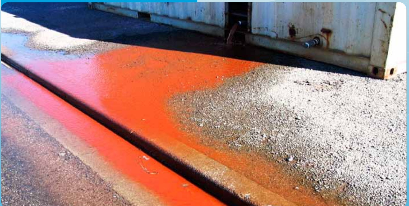
Rusty condensate water flowing into a gutter.
