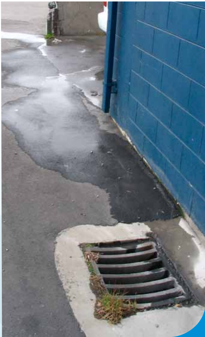
Run off from the car wash drains into the stormwater network.
