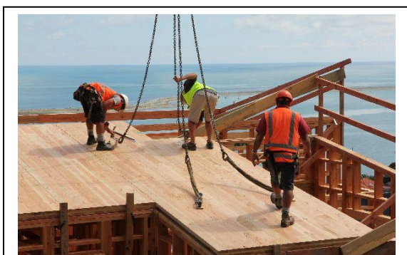
Figure 5.4 - CLRT panels used as flooring ( www.xlam.co.nz )
