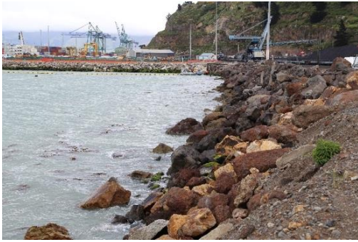
Figure 2 Section of stone riprap near the reclamation facing south after approximately 60 years of placement (with regular maintenance).
