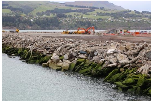
Figure 3 Existing temporary eastward face of reclamation (Nov 2016) after approximately 24 months of placement.
