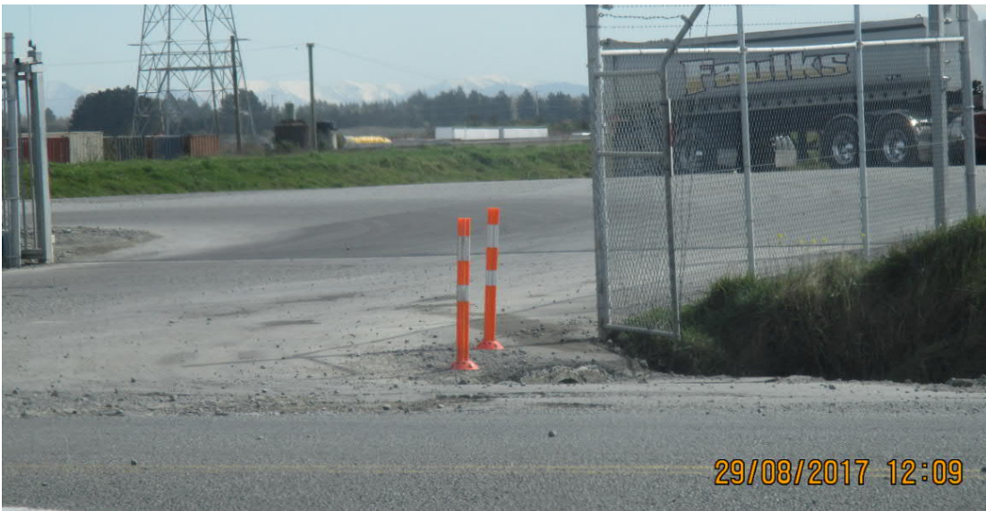
Photograph 2 - Road Metals access surface damage & loose chip - Council Compliance Unit 29/08/2017
