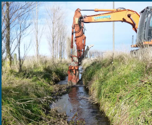
Image 3: Digger excavating trench in stream bed for weir installation
