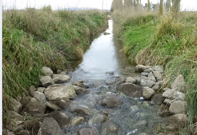
Image 2: Installed rock weir showing placement of boulders creating slight slope downstream and armouring of stream banks
