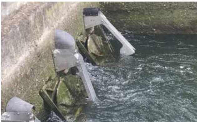
Modified floodgates at Courtenay Stream
