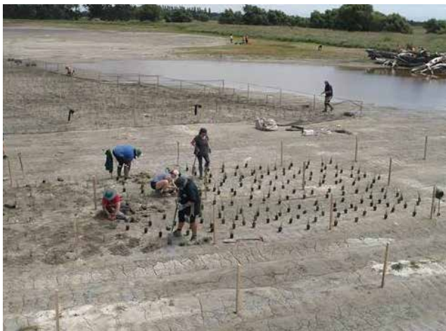
Installation of 80,000 aquatic plants at the Whakaora Te Ahuriri constructed wetland
