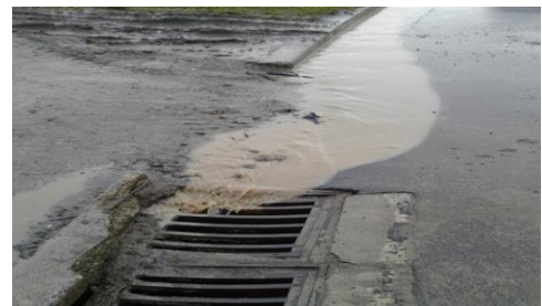
Photo 7: Sediment running into a stormwater drain
