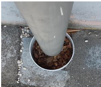
Photo 5: Blocked drain
