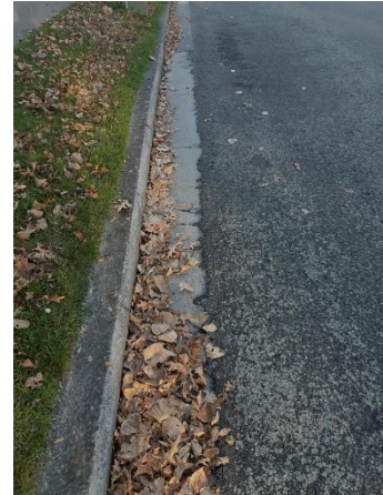
Photo 11: Although beautiful and fun to jump in these leaves can cause havoc with the stormwater network, clogging up drains and increasing the risk of localised flooding
