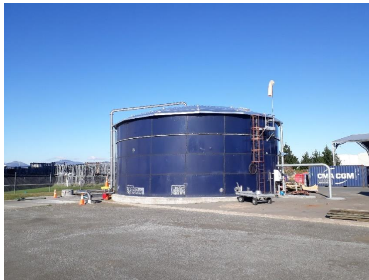
Figure 1: Effluent tank with lid installed
