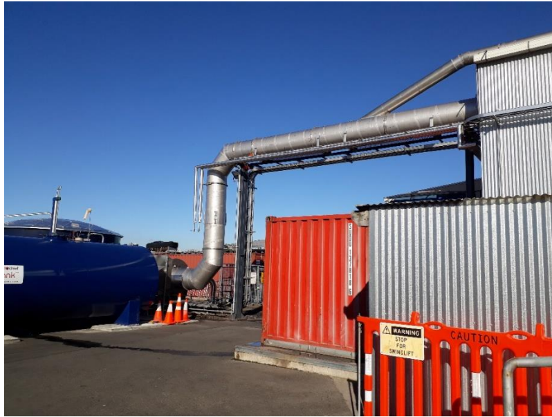
Figure 2: Upgraded ventilation / extraction system
