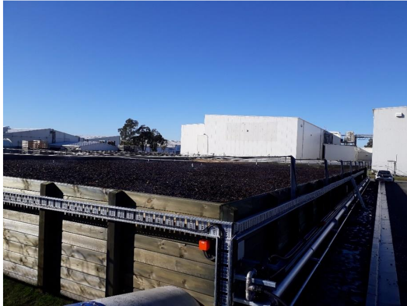
Figure 3: replacement bio filter
