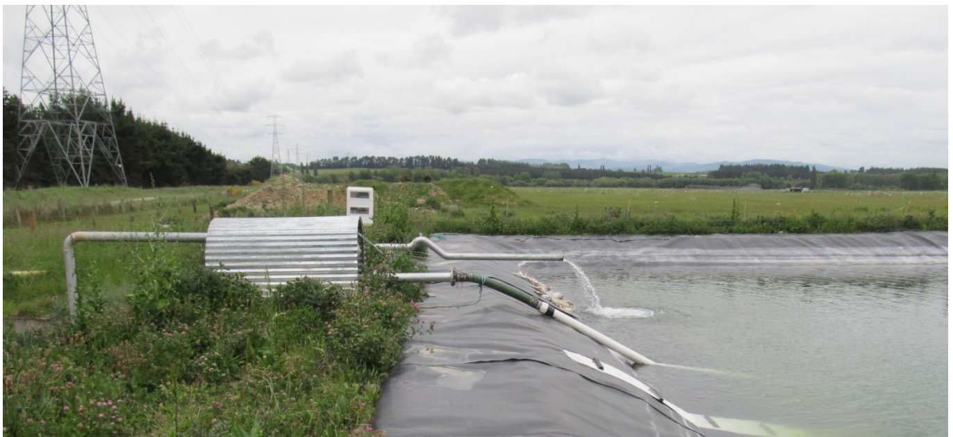
Fig 3: [taken 15-11-2015] The new pond. The base of the pond [in Figs 1 and 2] was filled in and then this new lined pond built over it, in its place. The combined flow of the three galleries goes through a flow meter (which send the relevant data to Ecan) and then enters the pond. [In front of this] water is extracted for irrigation. The Te Ngawai River is 1157M (Bob Hall's measurement – Ecan has it at 1200M) away – beyond the willows in the background. Looking North. Cross Rd on the left.
