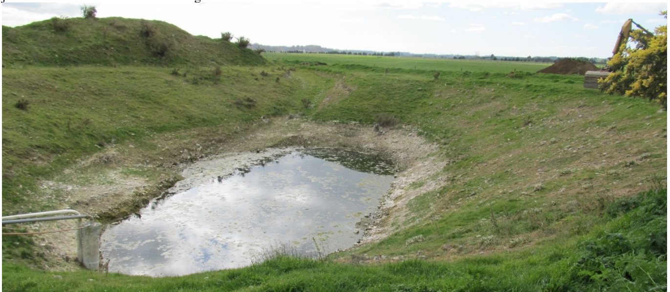
Fig 1: [Taken 9-9-2014] This is the set up I had up until this date. This is at the southern end of the first gallery I built (in 2001). The water flowed from the gallery into the pond. The white siltstone seen on the left-hand side is what occurs at the base of all the galleries. The water from the second and third galleries was added (the white pipe) and then the water used for irrigation was pumped out (the grey pipe) and spread using K-lines. The digger (right top corner) is about to make major changes.
